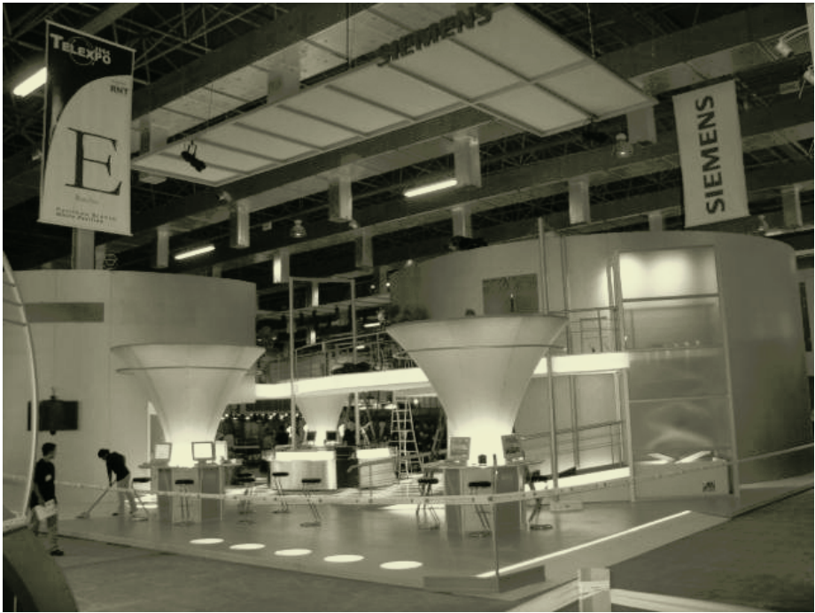
Fig. 5. Photo of the final stand being constructed at the fair site. This stand was considered the best in the fair
